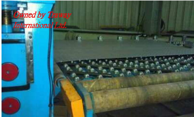
STEP 6 Checkered Plate was levelled horizontal
